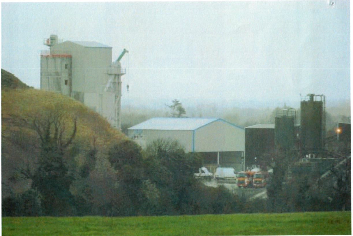
Construction of plant in 2016 without planning consent
